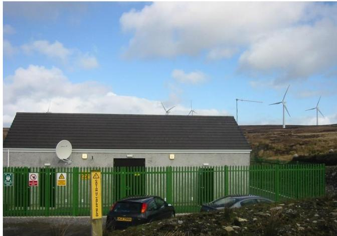
Substation connecting a wind farm into an electricity distribution network showing multiple terrestrial UHF and satellite radio links to monitor and control the associated switchgear.
