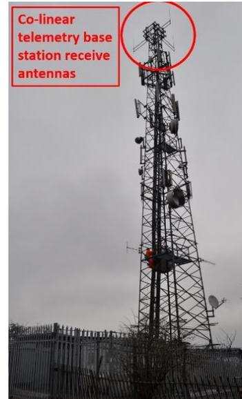
Typical high sited utility SCADA base station receive antennas in 460-470 MHz band.
