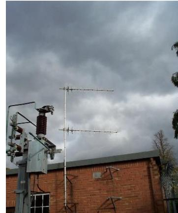
Typical Electricity substation antennas for SCADA outstation transmissions in 460-470 MHz band.
