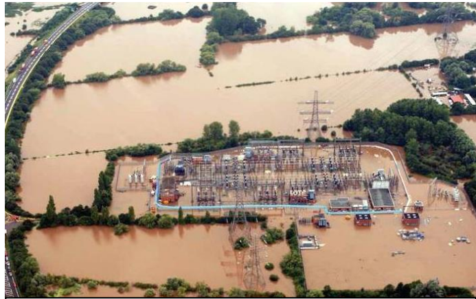
The Walham electricity substation inundated during the 2013 winter floods in the UK
