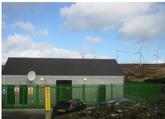
Substation connecting wind farm into an electricity distribution network showing multiple terrestrial UHF and satellite radio links to monitor and control the associated switchgear.
